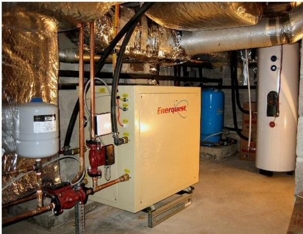
The heat pump provides both underfloor and forced air heating
