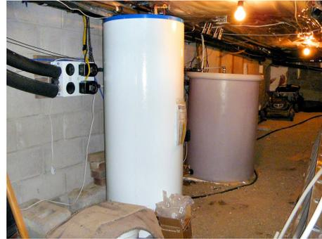
The cost of such systems is largely determined by the cost of the boreholes and ground heat exchangers. That cost can be minimized by installing buffers on the input and output lines of the heat pump. The buffers limit the temperature swing of the fluid in the exchange loop. Together with quad-tube ground heat exchangers these can reduce the capital cost of the ground system by as much as a factor of four and they will also reduce the amount of power needed by the heat pump.
