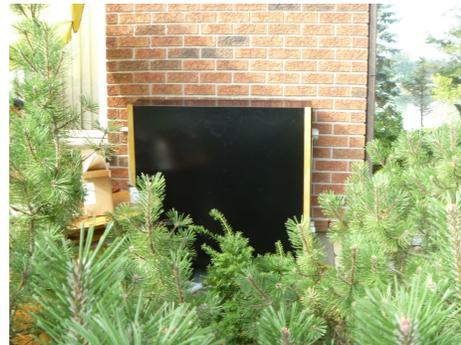
Buildings smaller than 100,000 square feet will commonly require a source of additional heat to be added to the ground store. The least expensive source of that heat is the summer air. Heat can be extracted from the air and transferred into the ground store to make up for any deficiency using an air heat exchanger like that pictured above.
