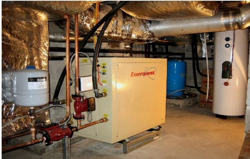
*The heat pump provides both underfloor and forced air heating*
